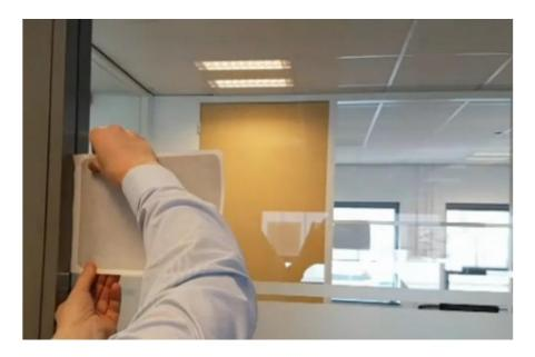
2) Place the foil with the desired size on the glass surface
